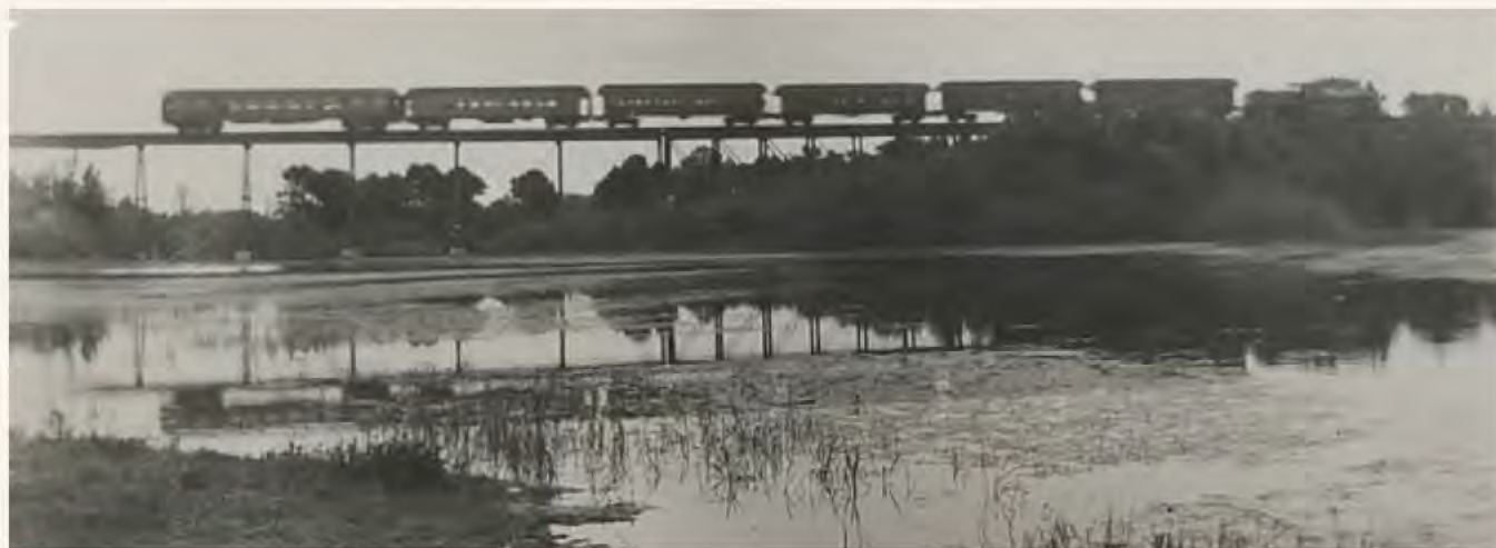
Figure 26 Photograph of first BCR&N railroad trestle north of Lincoln Street in Estherville. Courtesy of Emmet County Historical Society.
